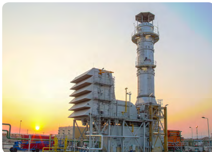
Fig. 1 – The First MGT-40 gas turbine installed at Zahedan power plant
